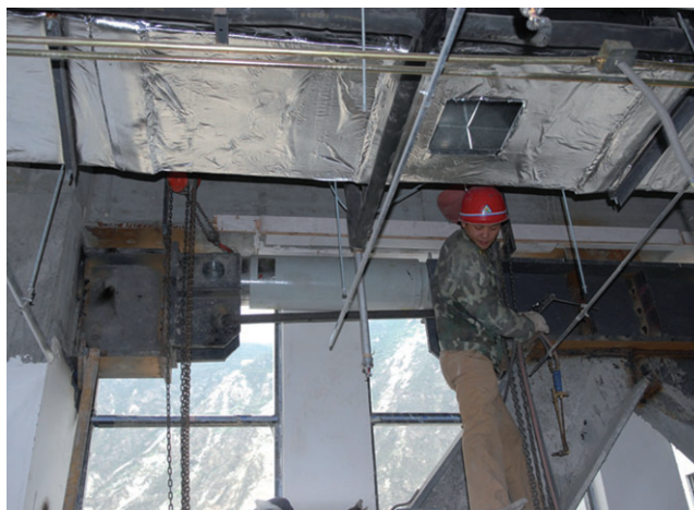
Figure 5. Installation of viscous damper
